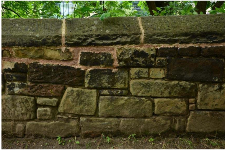
Ashlar Wall on Hume Walk
