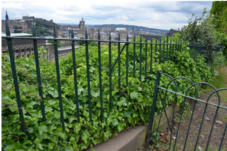
Bow Top and Spiked Fencing
